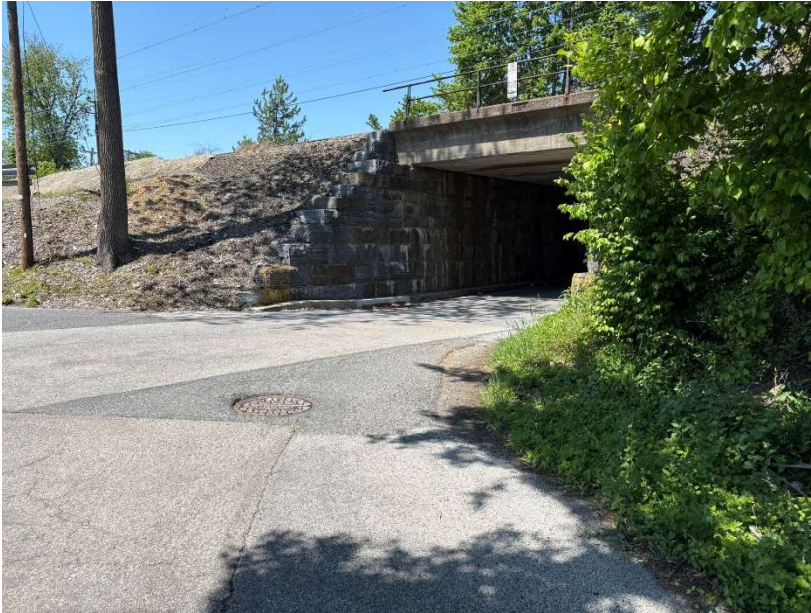
Lakeside Avenue stop-controlled approach looking right towards the rail line bridge
